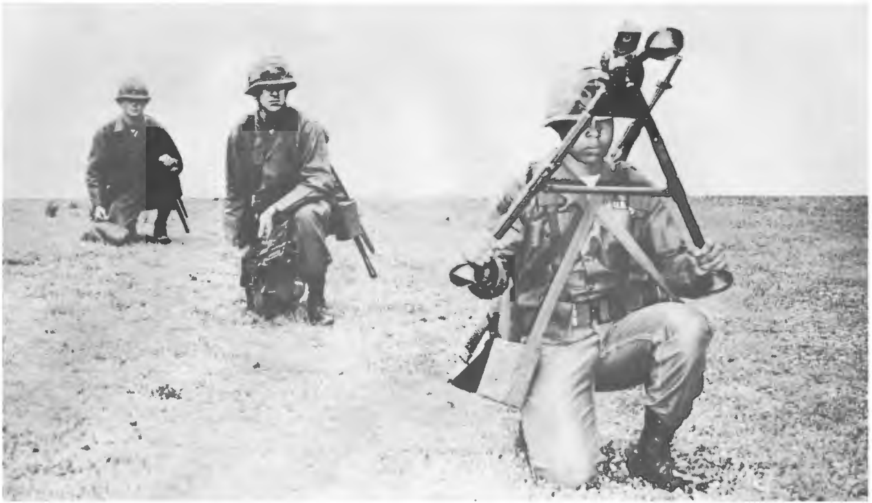
Figure 63. Opening the tripod.
