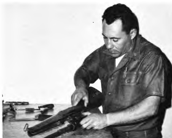
Figure 7-2.—Disassembling the weapon for cleaning.
